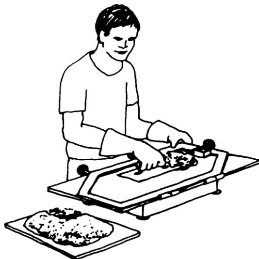
Figure 2: Work the mortar mix under vibration
